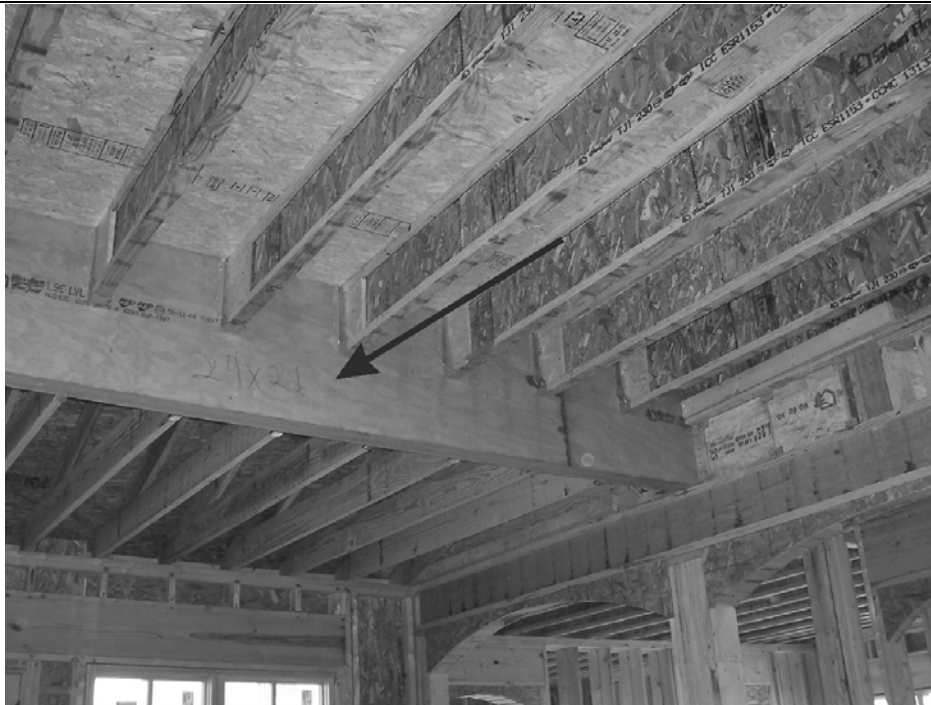
Figure P2603.2(7) LAMINATED VENEER LUMBER BEAM
