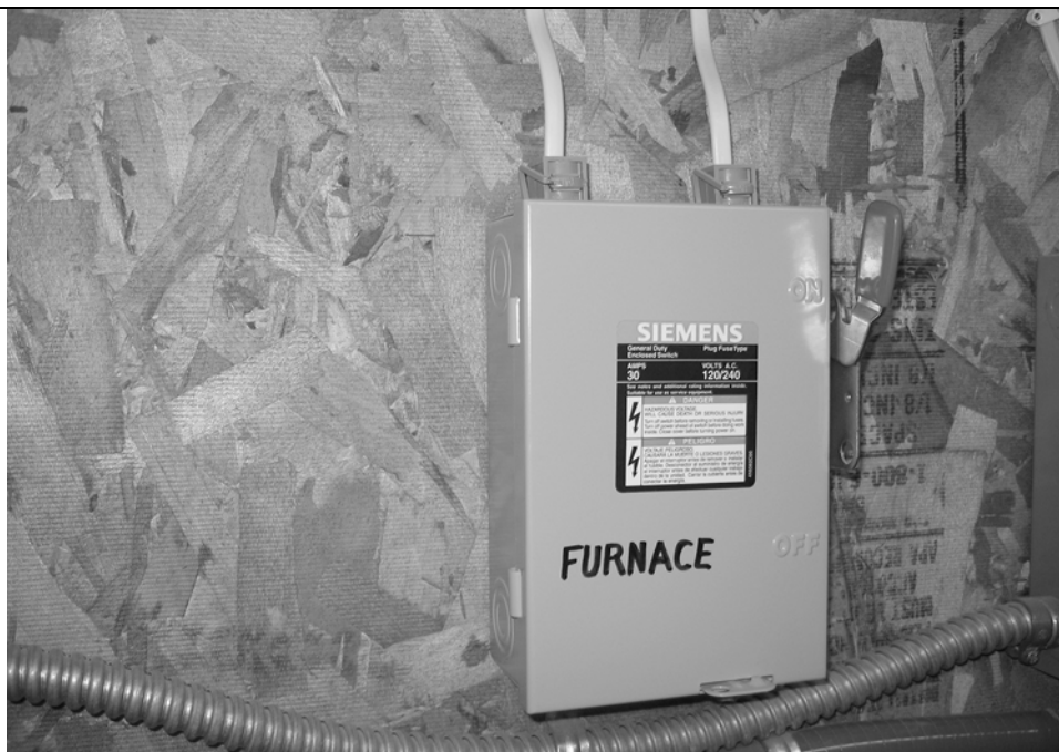
Figure E4101.5 TYPICAL APPLIANCE DISCONNECTING MEANS
