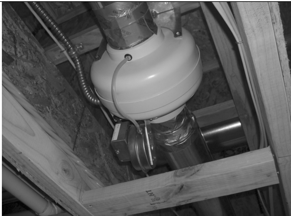
Figure M1502.4.4 DRYER EXHAUST DUCT POWER VENTILATOR
