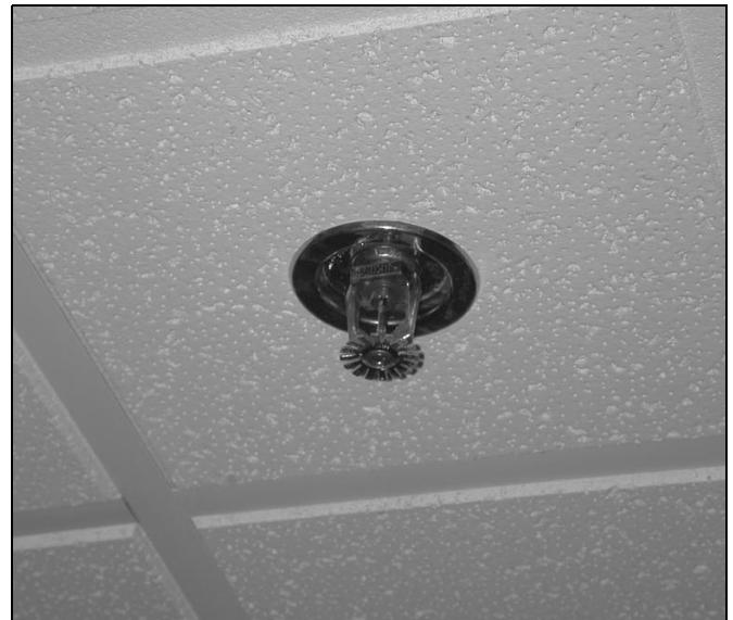
Figure P2904.2(1) PENDANT SPRINKLER
