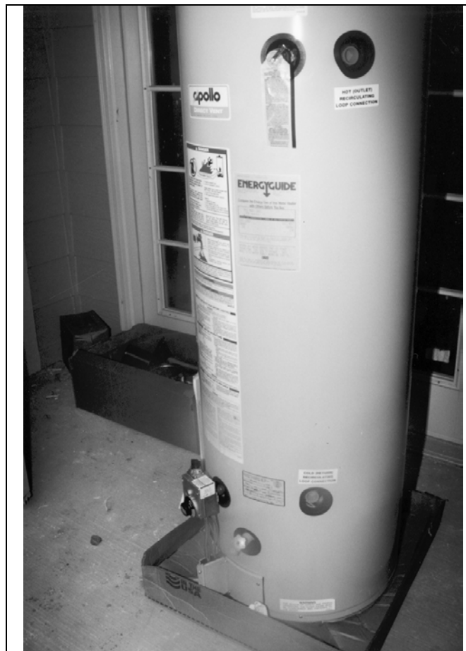
Figure G2448.2(1) DIRECT-VENT WATER HEATER DESIGNED FOR BOTH POTABLE WATER HEATING AND SPACE HEATING APPLICATIONS
