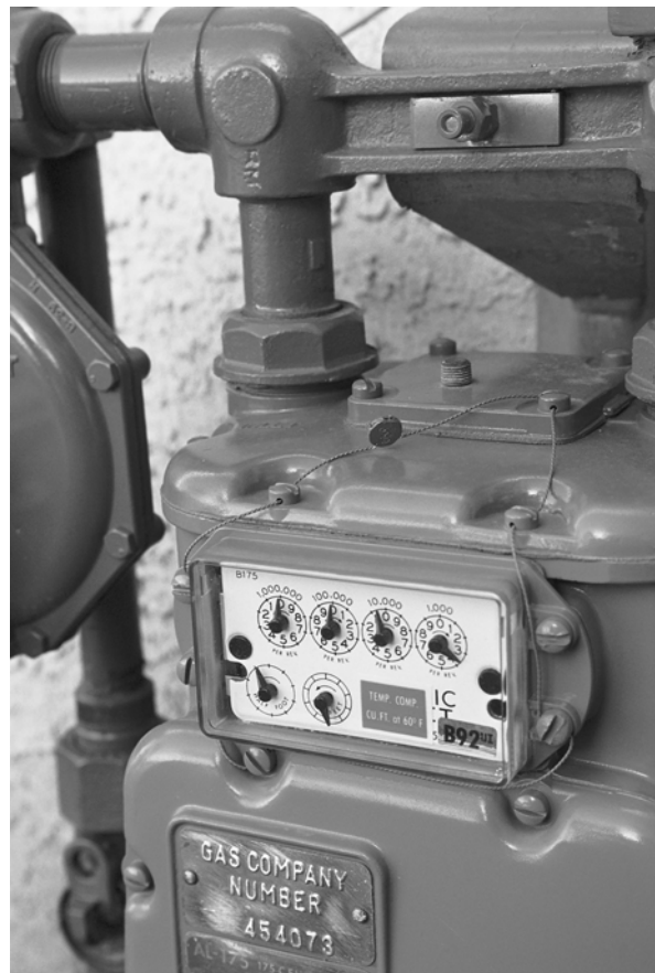
Figure 2414.10.4(2) OUTDOOR METER SETTING
