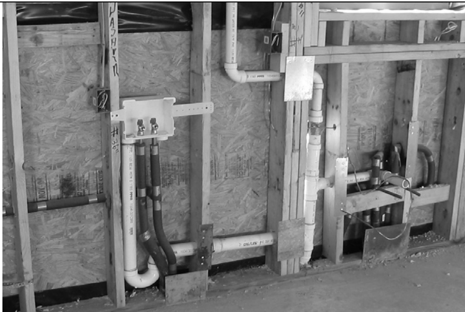
Figure P2603.5(3) PIPING IN EXTERIOR WALL
