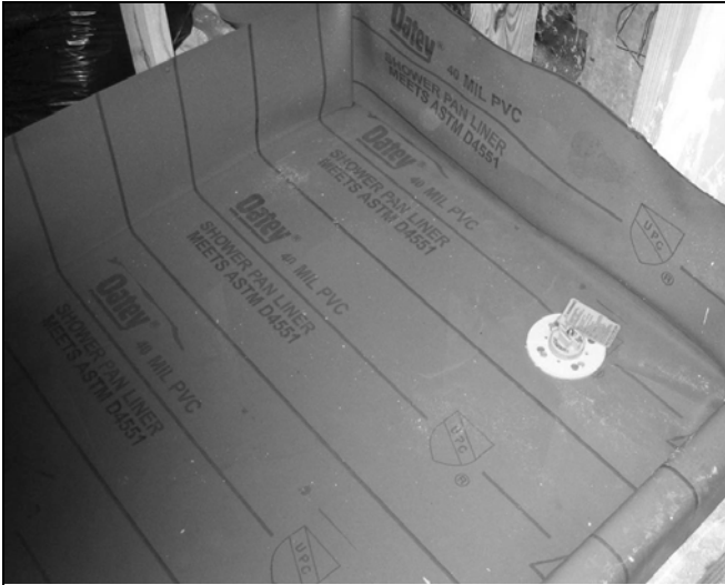
Figure P2503.6(2) INSTALLED SHOWER LINER READY FOR TESTING
