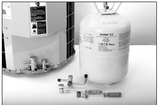
Figure M1411.8(1) INSTALLATION OF LOCKING CAPS FOR REFRIGERANT ACCESS PORT
