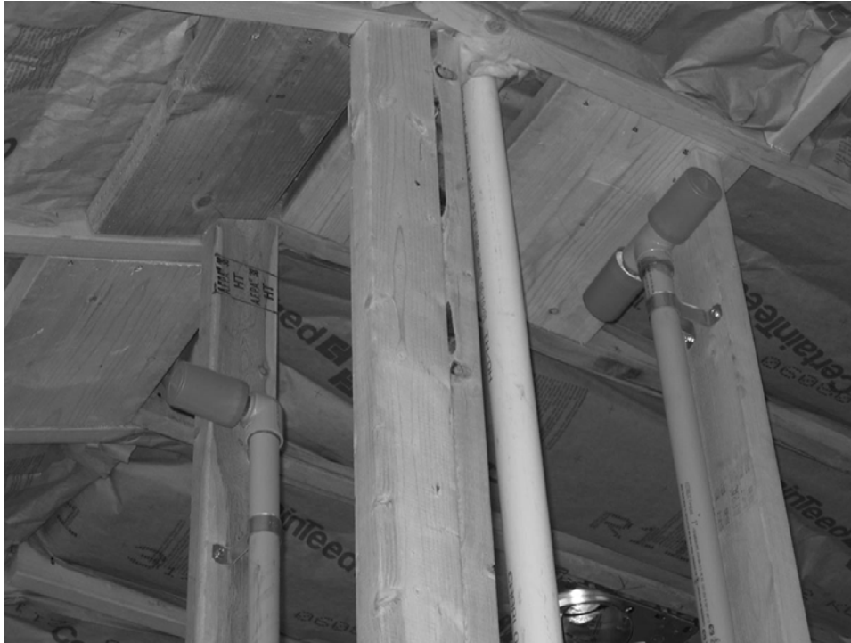
Figure P2904.8.1(1) SPRINKLER SYSTEM ROUGH-IN
