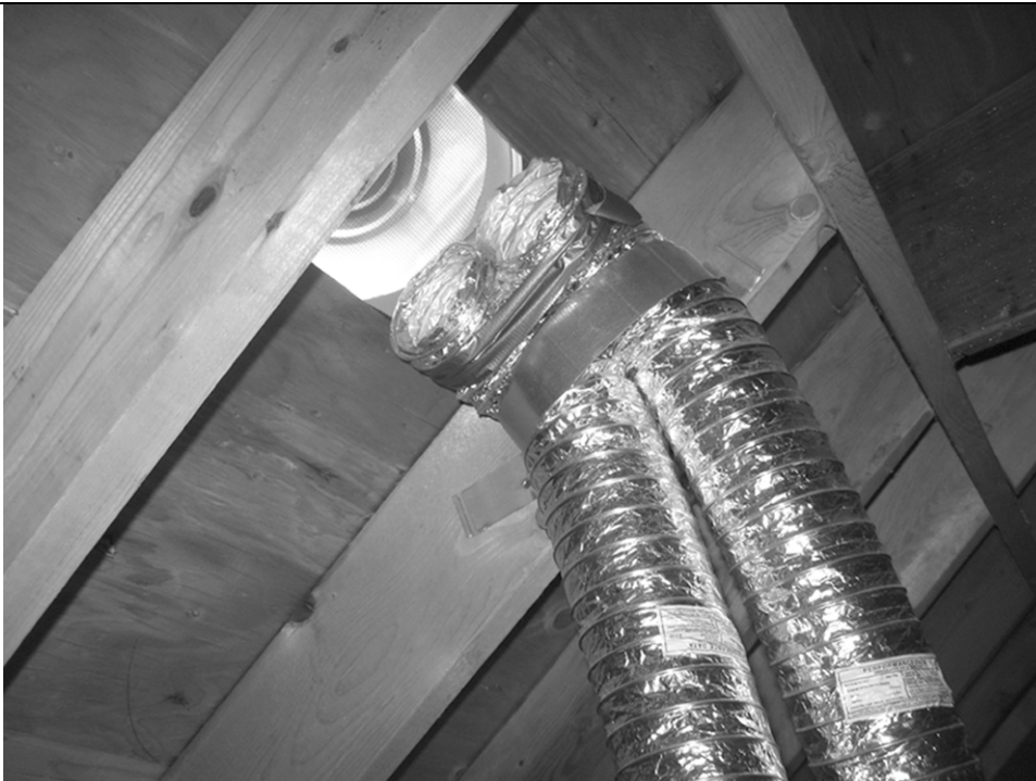
Figure M1501.1 PROHIBITED EXHAUST TERMINATION
