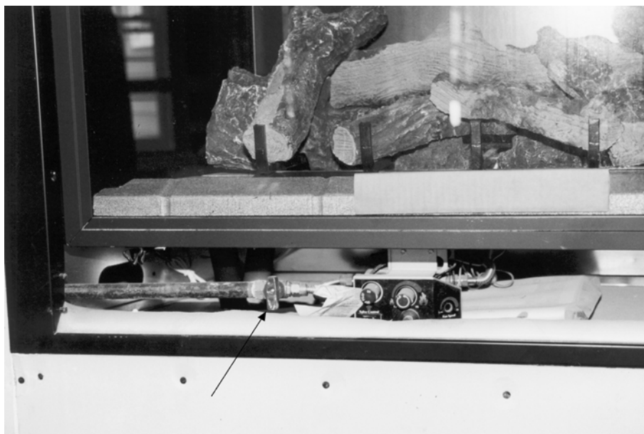
Figure G2420.5.1 SHUTOFF VALVE IN CONTROL COMPARTMENT OF GAS FIREPLACE
