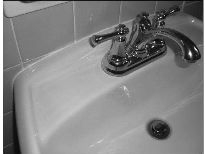
Figure P2705.1(2) LAVATORY PROPERLY SEALED TO WALL
