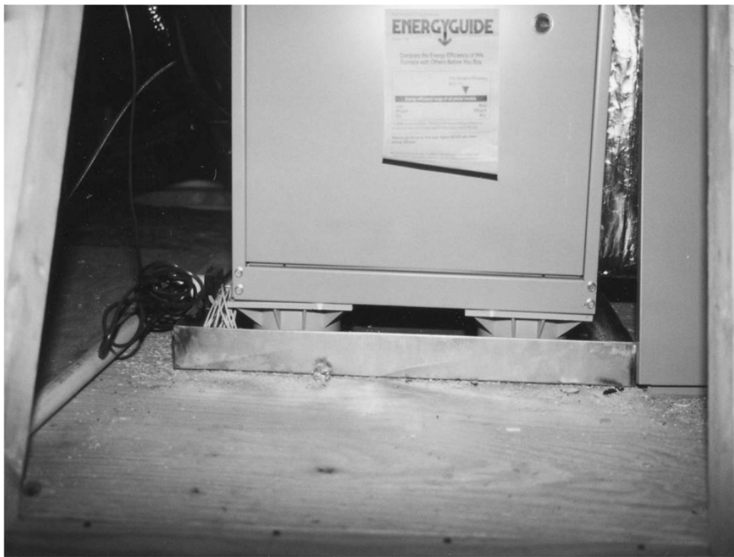
Figure M1411.3.4(2) ACCEPTABLE APPLIANCE AND PAN INSTALLATION
