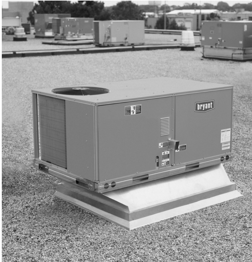
Figure G2427.2.2(3) ROOFTOP HVAC UNIT WITH INTEGRAL POWER VENT
