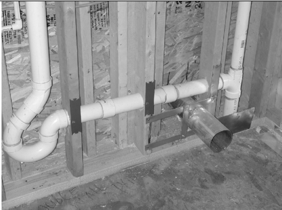
Figure M1502.4.7 SPACE FOR CLOTHES DRYER INSTALLATION
