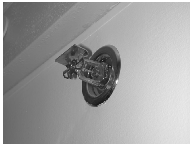
Figure P2904.2(2) HORIZONTAL SIDEWALL SPRINKLER
