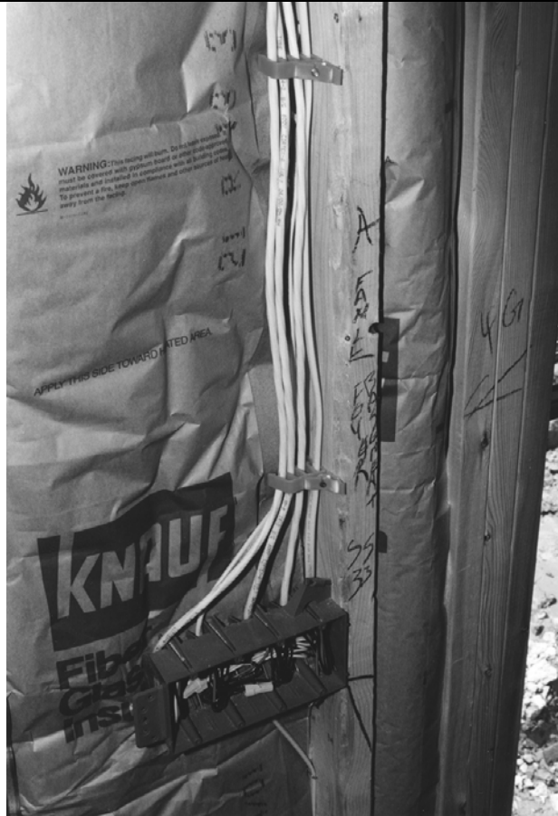
Figure E3802.1 CABLES HELD 1 1 / 4 INCHES BACK FROM EDGE OF FRAMING MEMBER
