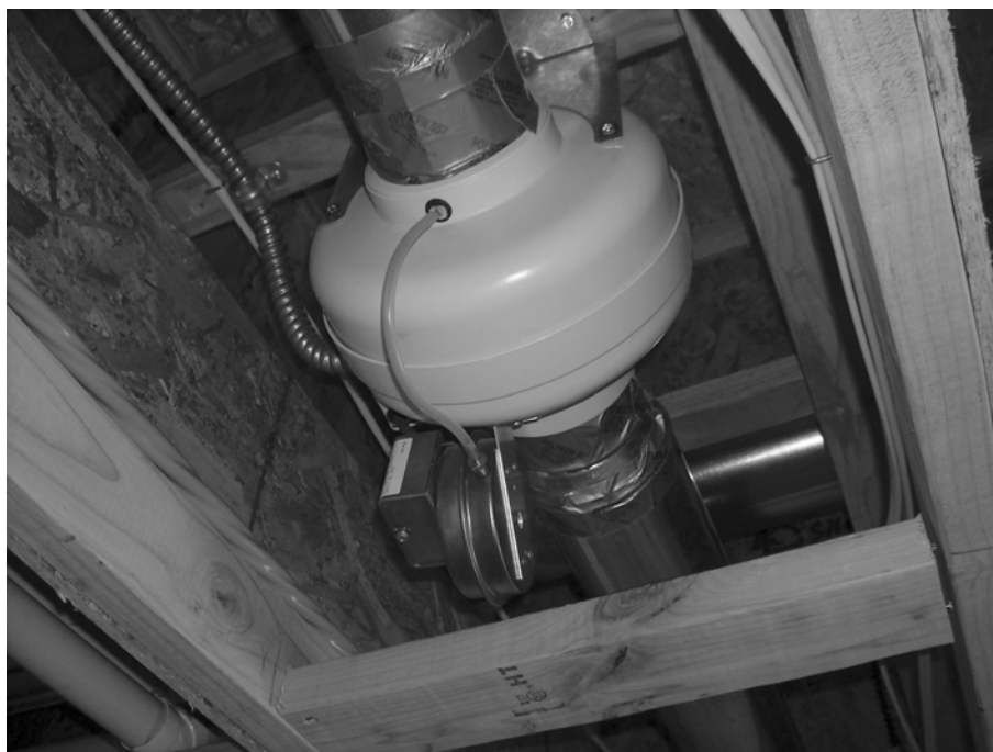
Figure G2439.4(1) DRYER EXHAUST DUCT POWER VENTILATORS
